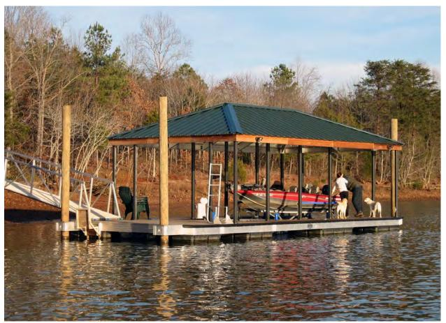
Figure 2. Example of Floating Pole Dock
