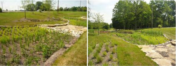
Figure 124. Bioretention Basins (stormwater.wef.org)
