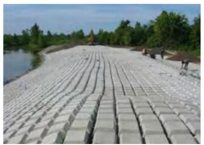
Figure 6. Example of Articulated Concrete Matting Erosion Control (iecsusa.com)
