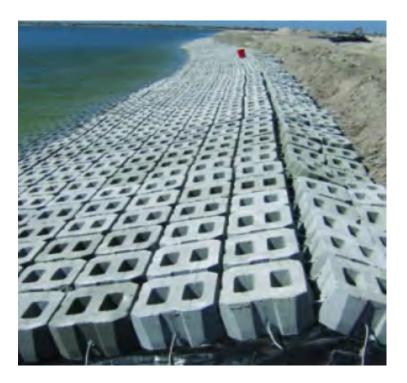
Figure 5. Articulated Concrete Blocks Example (Acfenvironmental.com)
