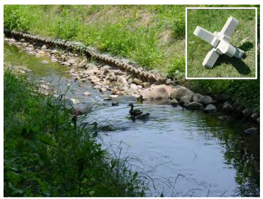
Figure 7. Example of A-Jack Revetment (conteches.com)
